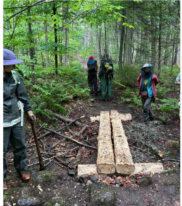
A finished, native-lumber bog bridge on Johns Brook Property
